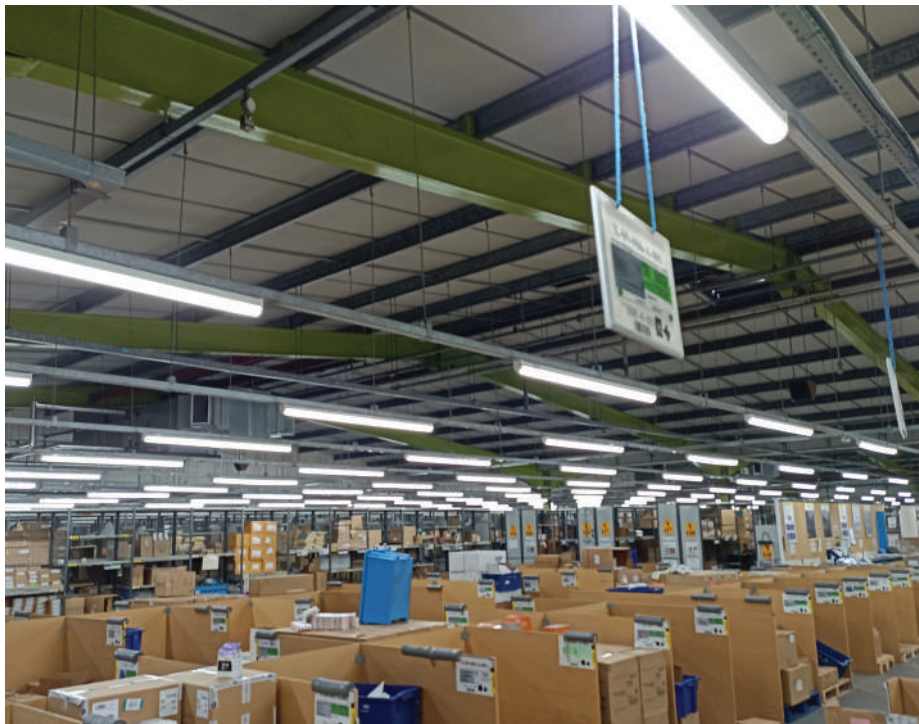
NHS Warehouse, Alfreton, UK
